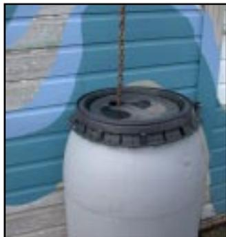
Drill a 7/8" hole 2 inches from the top of the barrel for an overflow vent hole. The hole can also be used to connect a second rain barrel. Additional rain barrels can be added to the assembly simply by using a double threaded pipe segment and appropriate hardware. Also, items such as a segment of garden hose and hose clamps can be utilized for the same effect. Use what you have!
